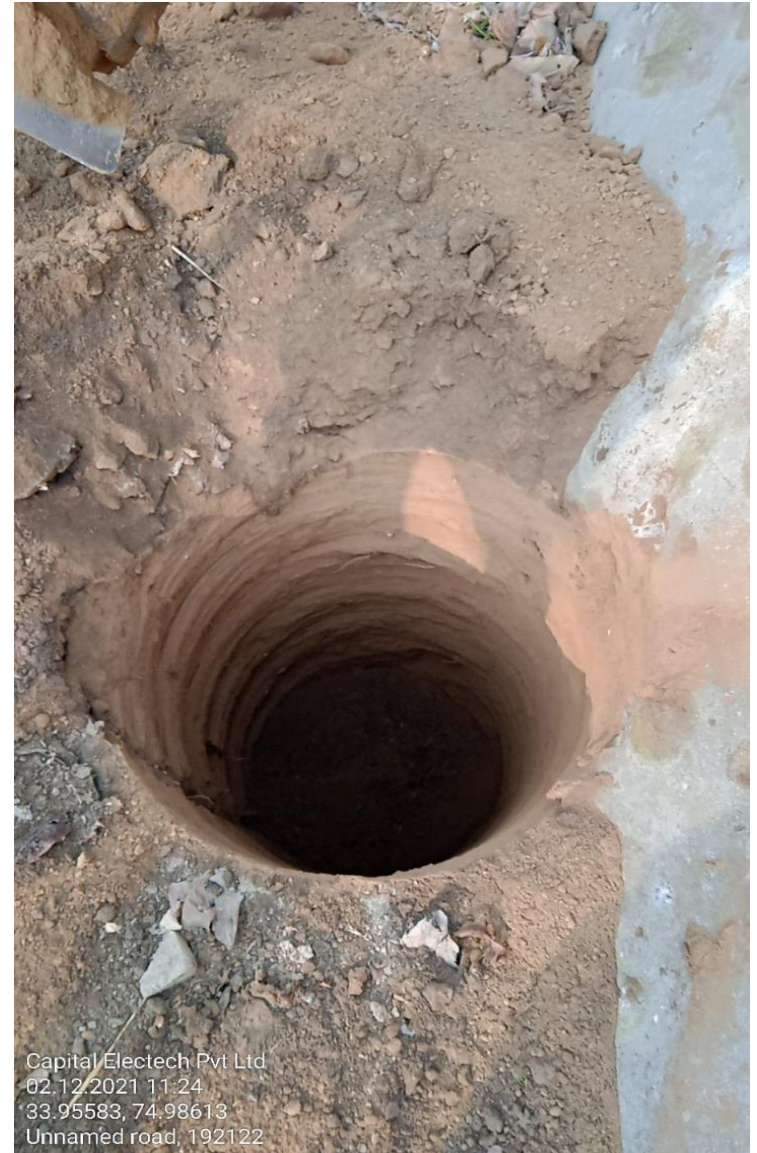
Installation of poles by mechanized means at Village Marhama in District Anantnag
