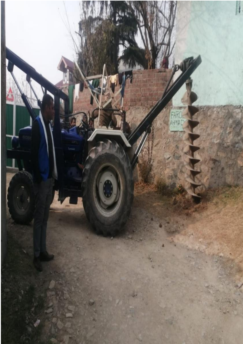
Installation of poles by mechanized means at Village Marhama in District Anantnag
